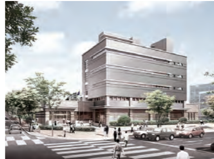
청주 지방검찰청 영동지청 Cheongju District Public Procurator's Office Building, Yeongdong Branch
