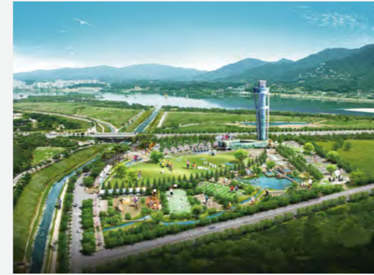
하남시 환경기초시설 현대화 및 공원조성사업 일괄입찰 기본설계 Preliminary Design for Wastewater & Waste Treatment Facility and Parks in Hanam 하수처리용량 : Q=32,000m 3 /일 중계펌프장 : Q=160,000m 3 /일(우수 80,000m 3 /일, 우수 80,000m 3 /일) 폐기물처리시설 : 음식물자원화시설 : 80톤/일(사료화) 소각시설 : 48톤/일(스토커식) / 재활용선별시설 : 50톤/일 압축장시설 : 60톤/일 / 적환장 : 4,500m 3 / 사업면적 : 81,020m 2 Public Wastewater Treatment Capacity : Q=32,000m 3 /day Relay Pumping Station : Q=160,000m 3 /day(Wastewater 80,000m 3 /day Rainwater 80,000m 3 /day Solid Waste Treatment : Food Resource Recovery Facility_80ton/day Incineration Facility_48ton/day Recycling Sorter Facility : 50ton/day, Compression Facility : 60ton/day Waste Storage Facility : 4,500m 3 , Project site area : 81,020m 2 대우건설 Daewoo Engineering & Construction Co., Ltd.
