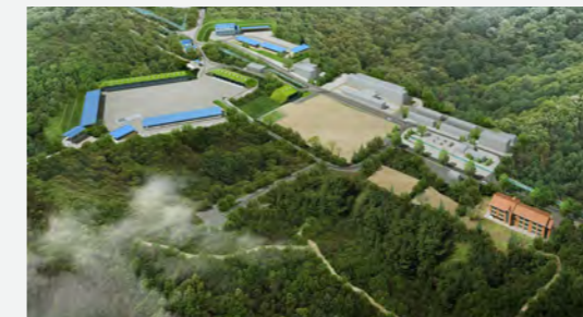
차기다련장3차 건설사업관리 Construction Management for Multi Launch Rocket System 3rd Related Facilities 연면적: 17,562㎡ 위치: 경기도 양주시, 동두천시 G.F.A: 17,562㎡ Location: Yangju, Dongducheon-si, Gyeonggi-do 국군재정관리단 The Armed Forces Financial Management Corps
